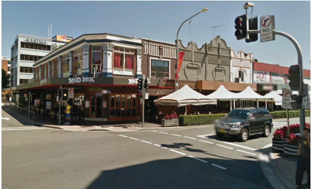
Figure 20: The group of shops at 281, 287, 289, 291 293 Church Street, listed on Schedule 5 of the Parramatta City Centre LEP (Items 74, 75, 76, 77 and 78)
