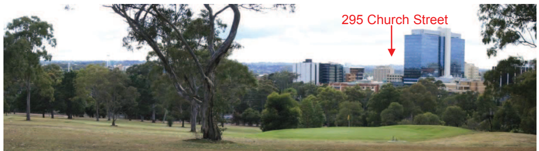
Figure 36: View 16 - approximate location of the subject site indicated
